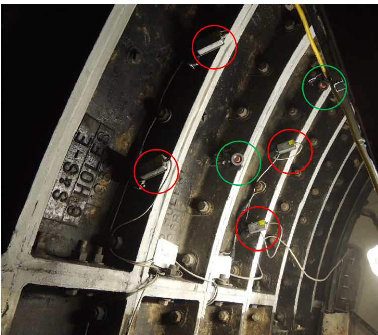
Fig. 9 Breakout tilt meters (red), optical targets (green).
