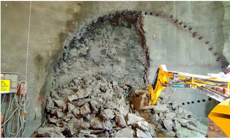
Fig. 8 Breakout of Adit tunnel top heading.
