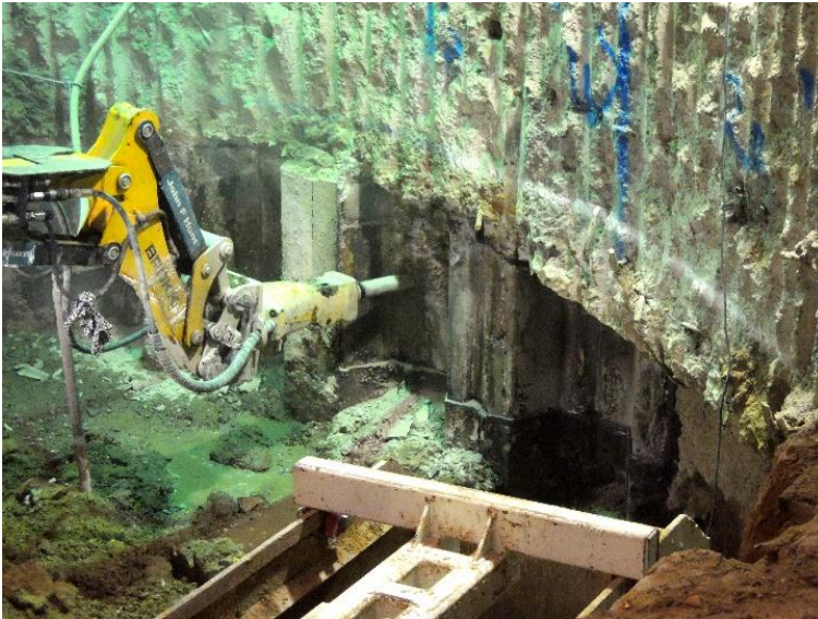
Fig. 6 Sheet piles exposed beneath structural slab.
