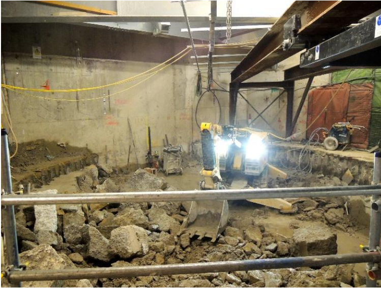
Fig. 5 Gantry crane installed above the SCL shaft.
