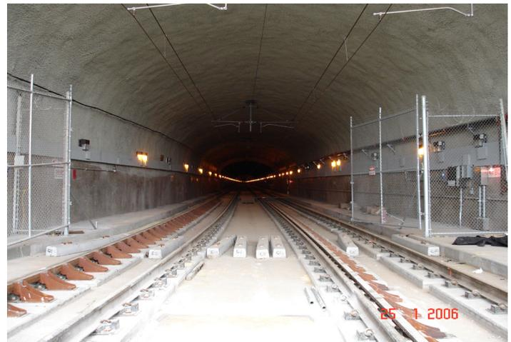
**Figure 2.** Finished transition into mined tunnel at the East Portal.
