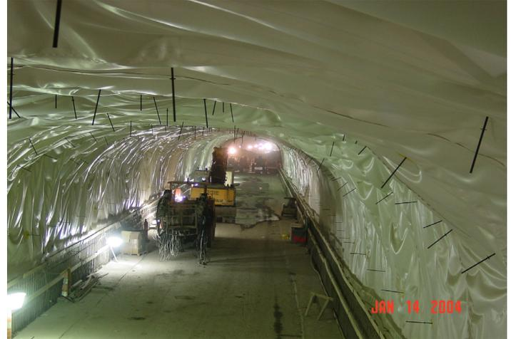
**Figure 1.** Membrane waterproofing system & BA anchors installed prior to secondary shotcrete final lining (SFL) installation in the transition section.
