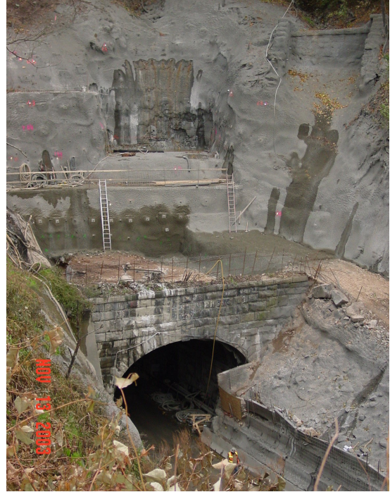
Figure 1. Existing portal and the construction of portal wall support.
