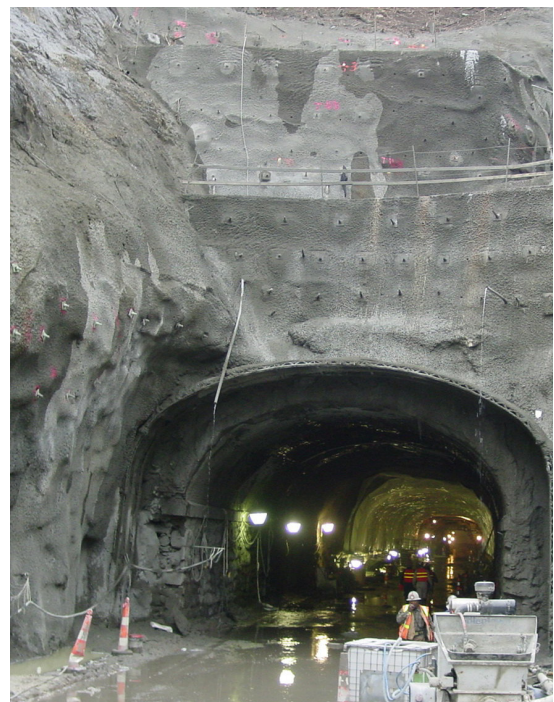
Figure 2. Shotcrete canopy construction for extension of the West Portal.
