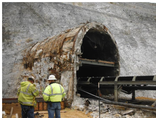
Figure 5: C6 Tunnel, partially unearthed during open pit mining activity
