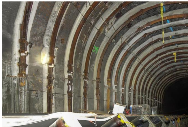
Figure 8: Completed tunnel section with TH steel sets
