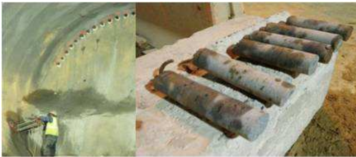
Fig. 11 Shotcrete strength test cores
