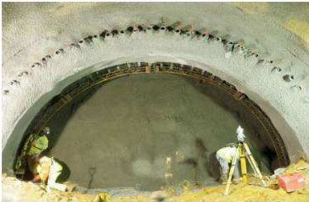
Fig. 8 Positioning the steel lattice girders in top heading and invert
