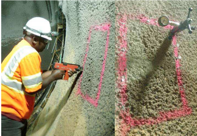
Fig. 10 Hilti Stud Driving Test
