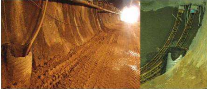
Fig. 6 Sump pumps installed in invert for dewatering
