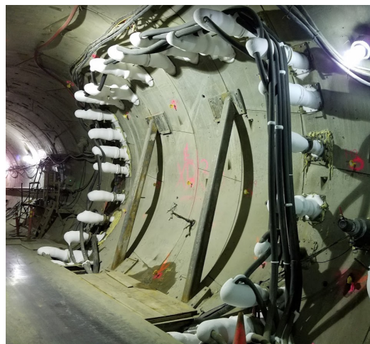
Figure 3. Ground freezing from inside the TBM tunnel
