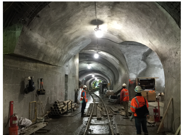
Figure 9. Cross passage fishmouth interface at the GCT 4 Facility
