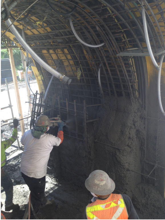
Figure 5. Pre-construction field trial PAC mock-up hand spraying of vertical walls
