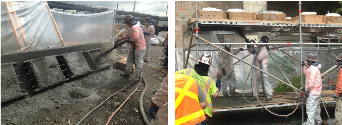
Figure 4. Preconstruction vertical (a) and overhead (b) test panels
