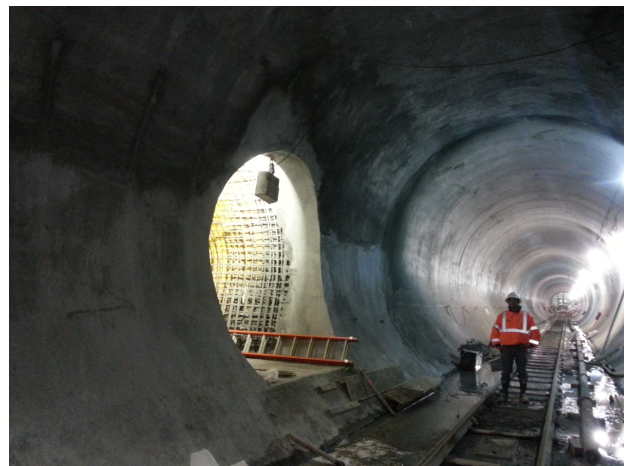
Figure 7. The fish mouth of a running tunnel cross passage (a) before and (b) after PAC application.
