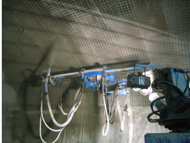
Figure 2. Typical Shotcrete Final Lining installation (Weehawken Tunnel in New Jersey, ca. 2004)
