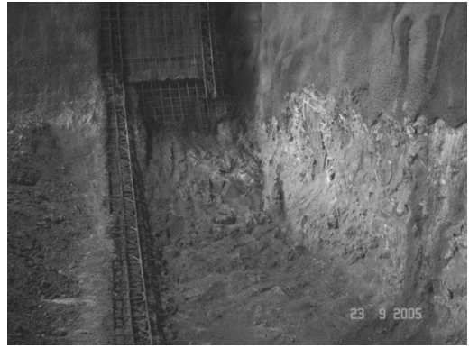
Figure 10. Invert excavation.
