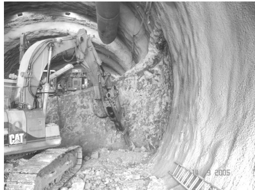
Figure 9. Bench excavation.
