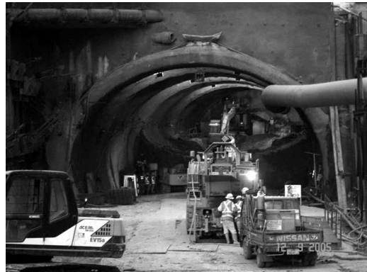
Figure 1. Fort canning tunnel.
