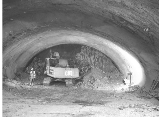
Figure 8. Top heading excavation.
