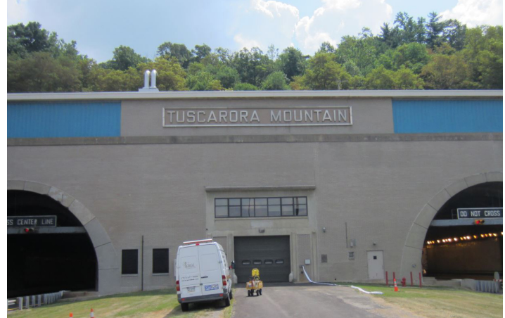
Figure 1. Tuscarora Tunnel Portal
