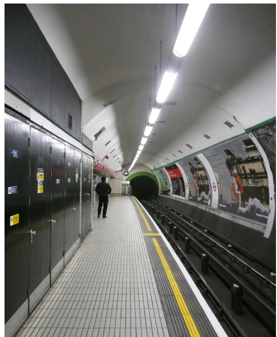
Figure 2. Interior of Tottenham Court Road Station.
