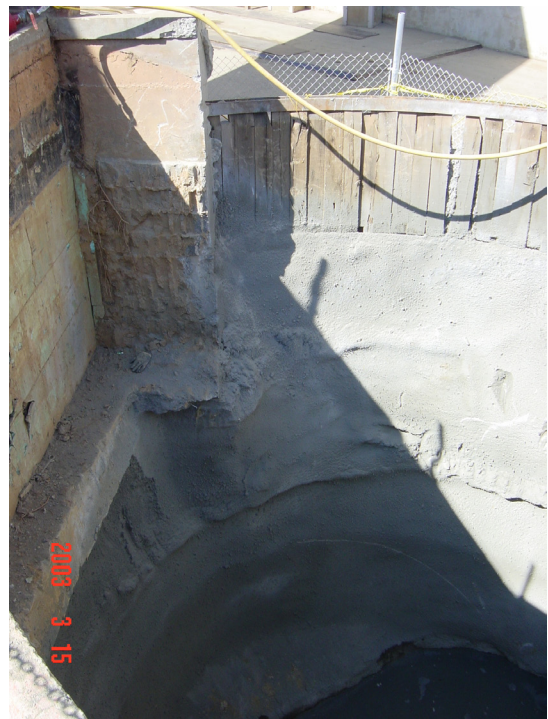
Figure 2. Shotcrete lined shaft and underpinning.
