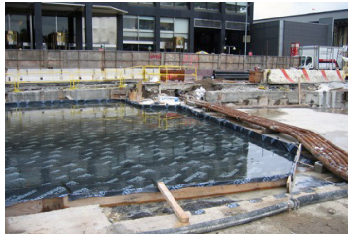
Figure 2. Waterproofing placement on structural box roof. (Courtesy of MTACC)
