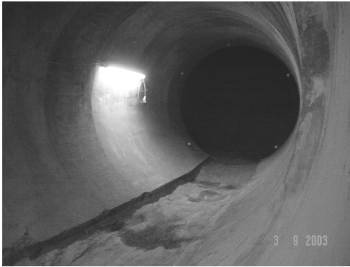
Figure 1. Trowel finished shotcrete lining.
