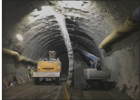
Figure 5. Excavation in left drift and preparation for setting girder in right drift
