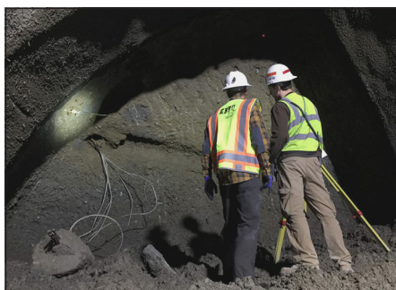
Figure 12. A tieback encountered during excavation next to Skyline basement
