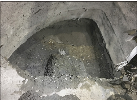
Figure 8. Face wedge formed during tunnel excavation under the utility trench
