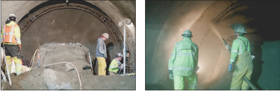
Figure 6. Lattice girder and shotcrete installation at the top heading
