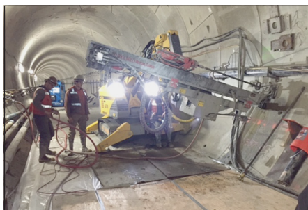
Figure 4. Ground probing from inside of the TBM tunnel
