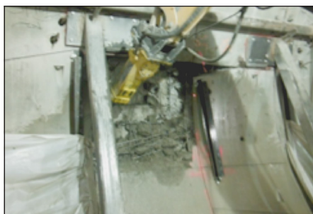
Breaking upper left segment
