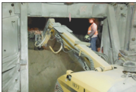
Excavating after removal of segments
