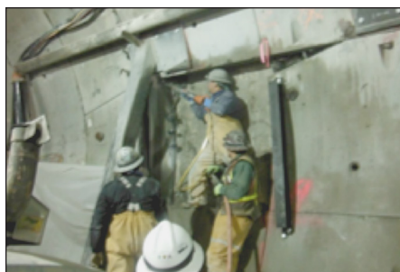
Removing rebar and bicone dowels
