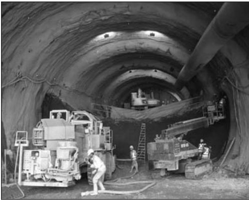
Figure 10. Fort Canning tunnel construction
