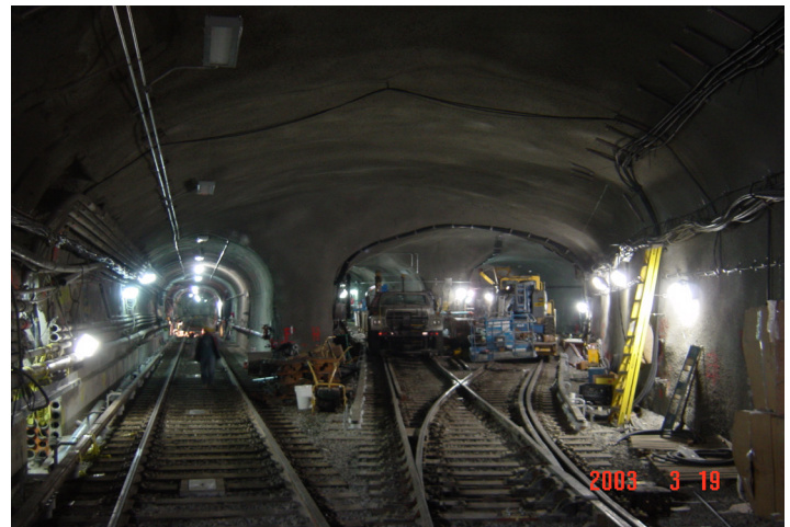
Figure 2. Station upgrade with enlargements constructed using shotcrete for the final lining.
