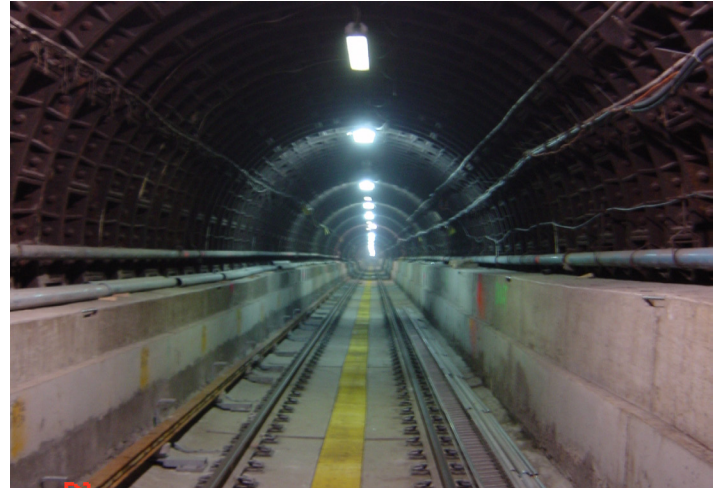
Figure 1. Rehabilitation of the PATH Systems Tunnel 'E'.
