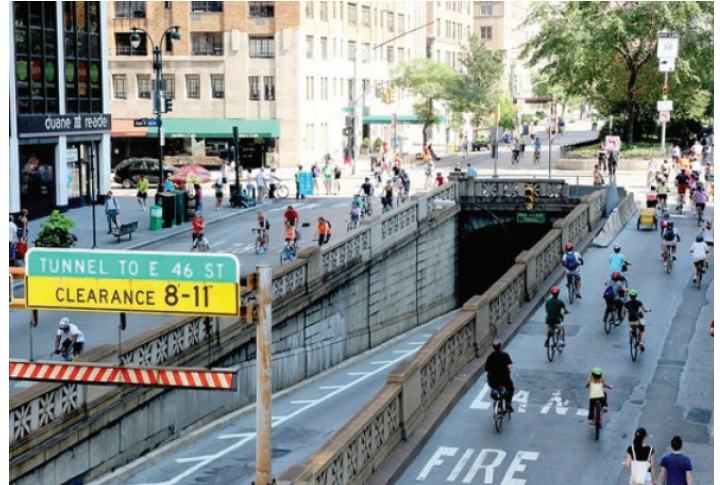
Figure 1. Park Avenue Tunnel, Image Courtesy of the DOT
