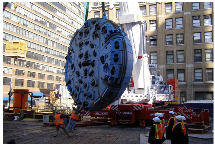
Figure 2. TBM cutter head being lowered into main shaft located in Manhattan.
