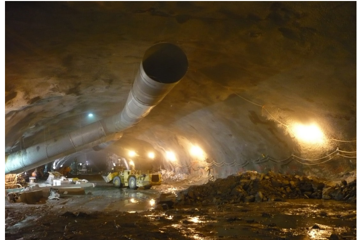
Figure 1. Station cavern after top heading and bench 1 excavation and support.
