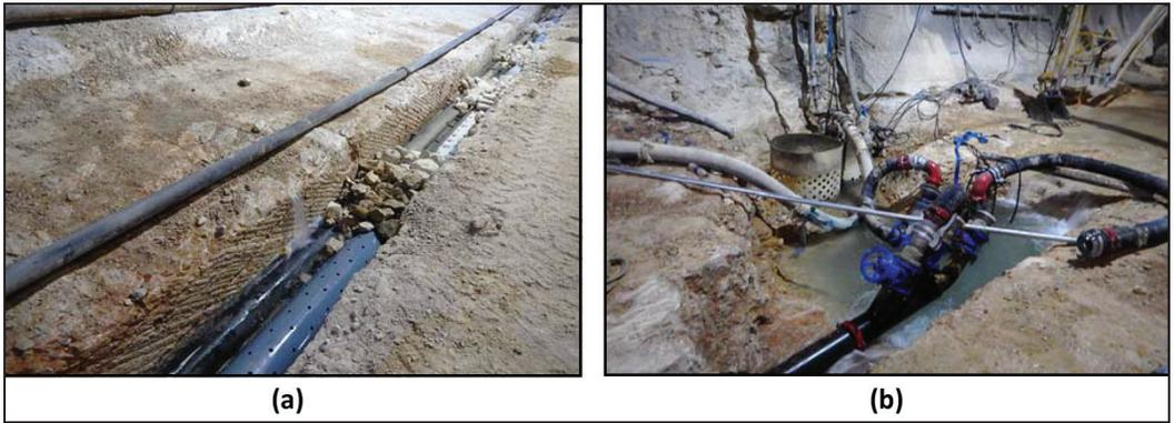
Figure 9. In-tunnel groundwater control: (a) trench with inlet and outlet piles, (b) temporary sump
