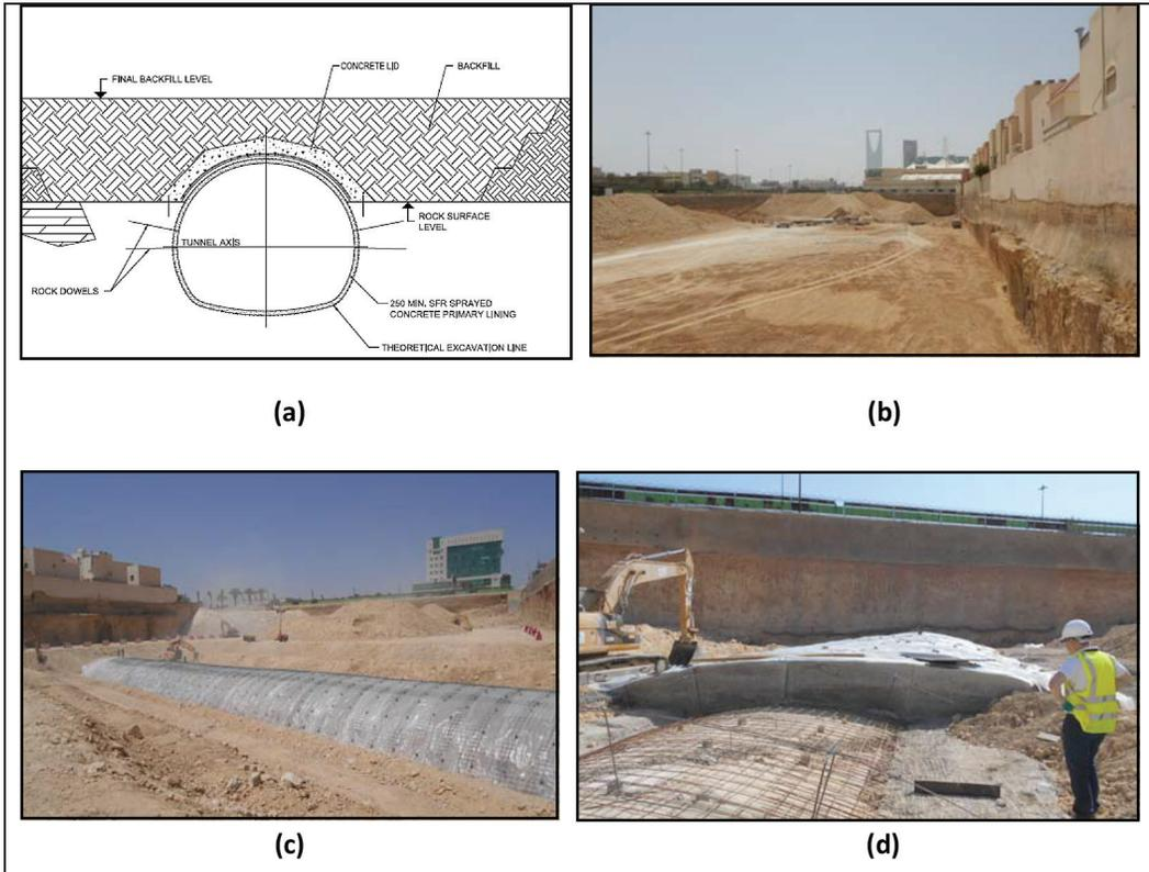
**Figure 8. Construction of west tunnel section within the open cut area: (a) tunnel configuration with respect to backfill and canopy lid, (b) open cut area before tunnel excavation, (c) backfill with PVC above the tunnel section, and (d) tunnel concrete canopy**
