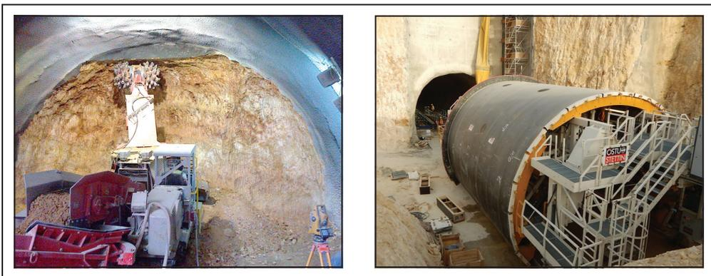
Figure 6. Tunnel excavation with roadheader (left) and secondary lining formwork (right)
