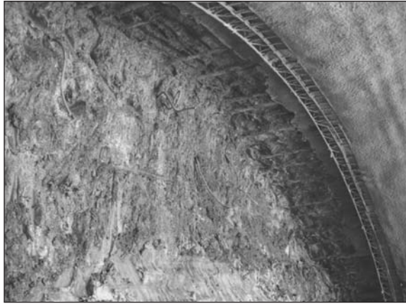
Figure 9. Top heading face shortly after excavation with exposed pre-support pipes
