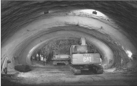
Figure 7. Initial shotcrete tunnel support in top heading
