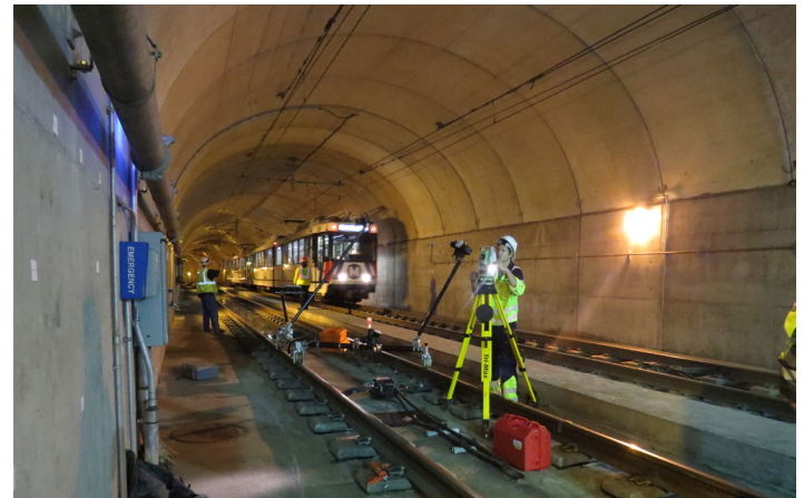
Figure 1. Digital Scan of Tunnel #3 During Detailed Inspection
