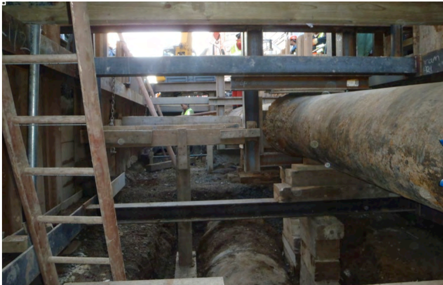
Figure 1 Some utility mains exposed beneath street level
