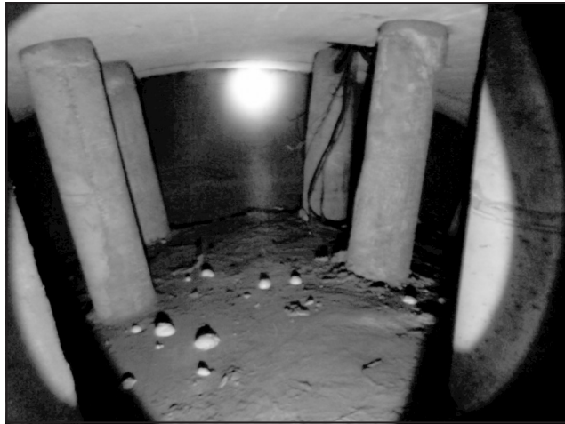
Figure 4. Embedded hangers in existing void space between main tunnel and ventilation arch wall
