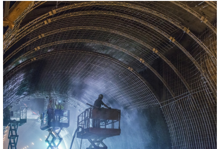
Figure 2. Preparation of a Center Arch section.
