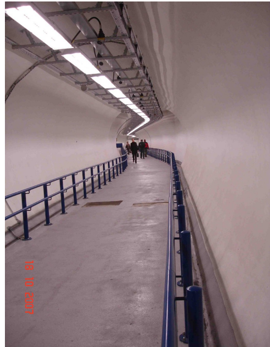
Figure 2. Temporary spur tunnel with shotcrete single pass lining.
