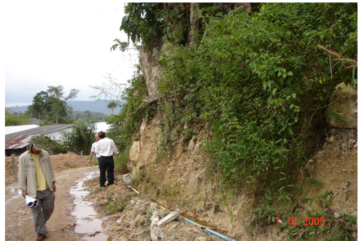
Figure 2. Contact zone between granite and sedimentary rock in East Portal area.
