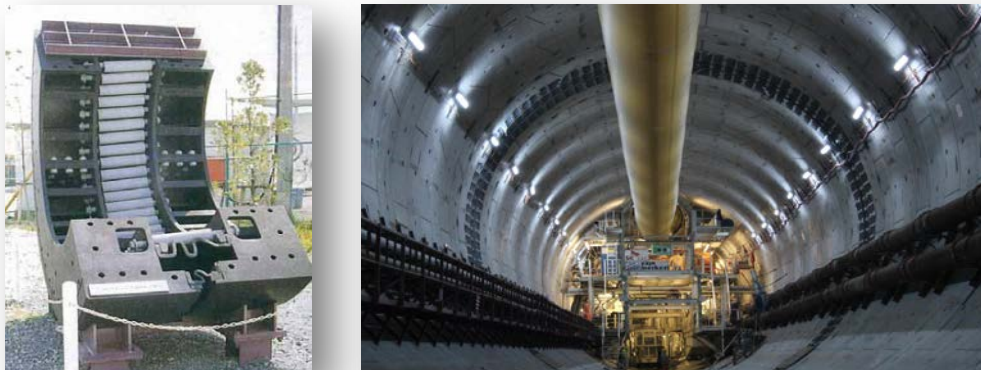
Figure 11 – Seismic Joint model and the joint in place
