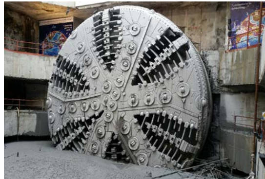
Figure 12 – TBM breakthrough
