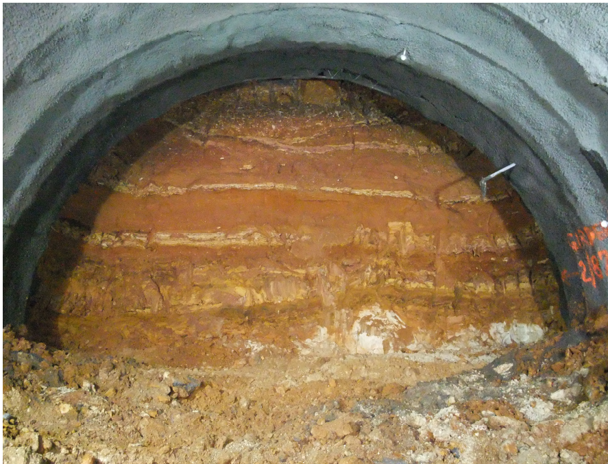
Figure 3. Outbound Tunnel Top Heading showing Interlayered Coastal Plain Sediments
