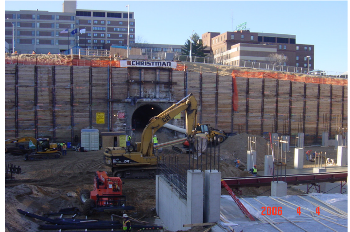
Figure 1. Entrance portal through support at excavation wall.
