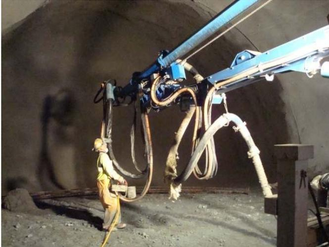
Fig. 2. Operator shown controlling the nozzle boom of the Meyco Potenza Shotcrete Robot utilized at Devil's Slide Tunnel.
