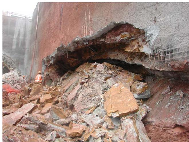
Figure 12: Localised failure along a bedding plane when a double-height bench was excavated.
