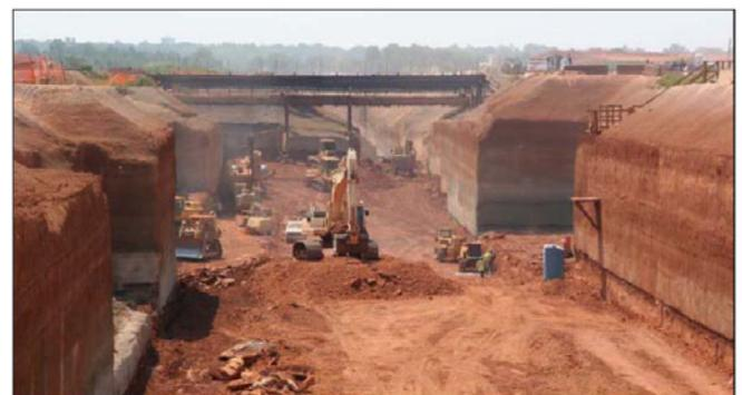
Figure 11: Typical rock cuts at Dulles Airport site (Tier 3 Excavation, photo from McQuinn et al 2006)
