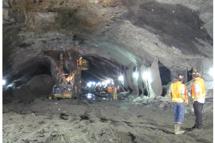
Figure 1. West-bound GCT Cavern arch rock bolt installation.
