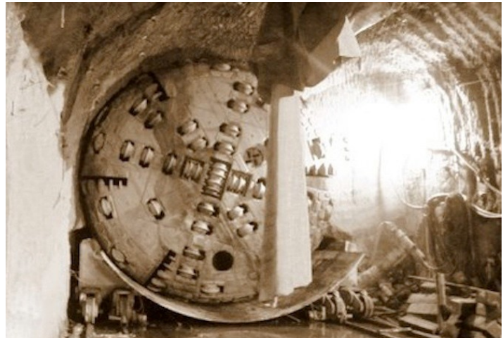
Figure 2. TBM emerging into Crossover Cavern. (Courtesy of MTACC)
