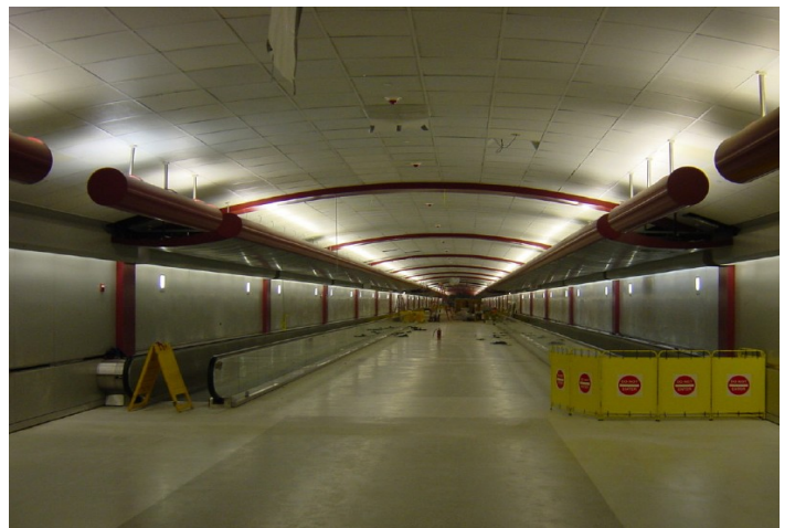
Figure 2. Installation of architectural finishes on moving walkways in the pedestrian tunnel.
