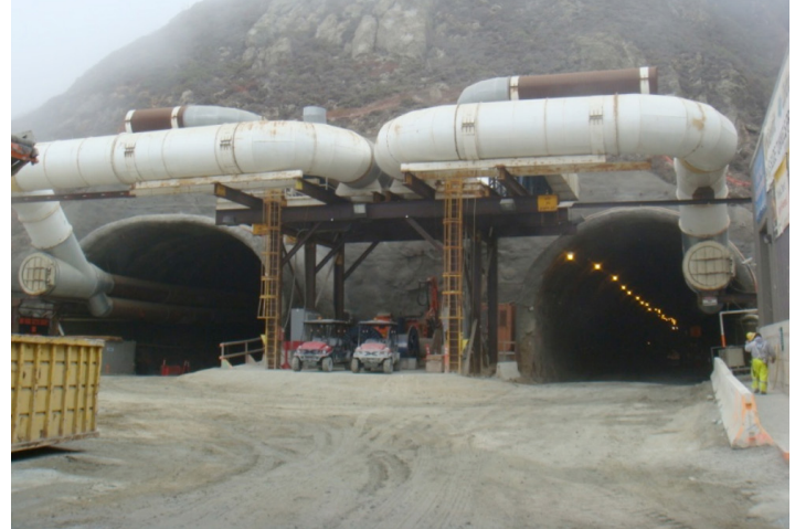
Figure 1. South portal during construction.
