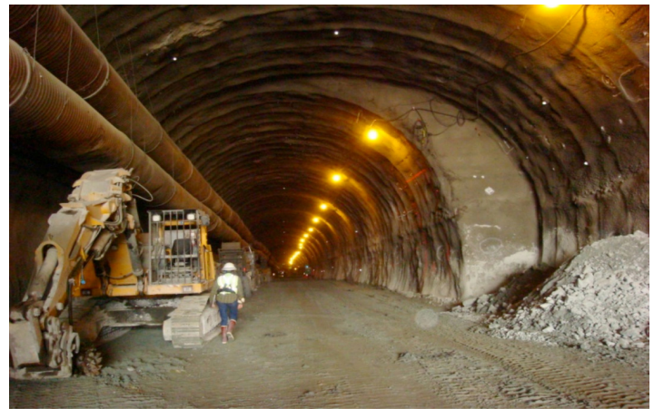
Figure 2. Southbound tunnel initial support.
