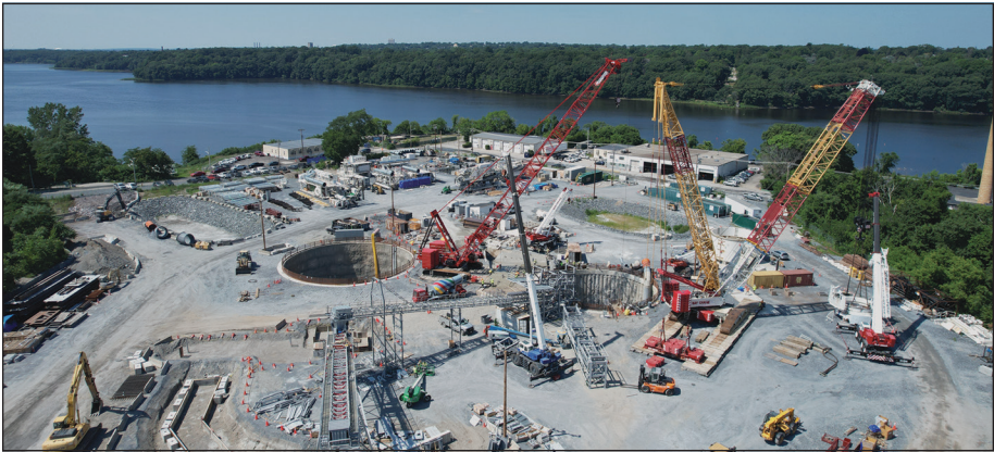
Figure 7. Main site aerial picture during TBM assembly
