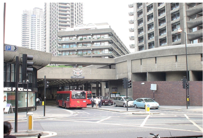
Figure 3. High-rise building along tunnel alignment.
