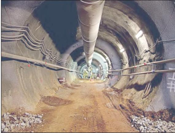
**Figure 5. View of inbound tunnel displaying sawteeth**
