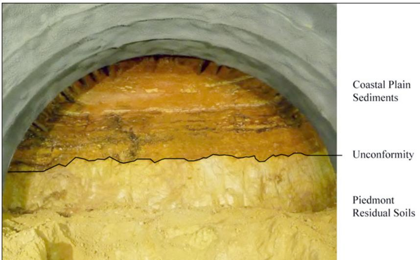
Figure 7. Coastal Plain sediments sitting unconformably atop Piedmont residual soil
