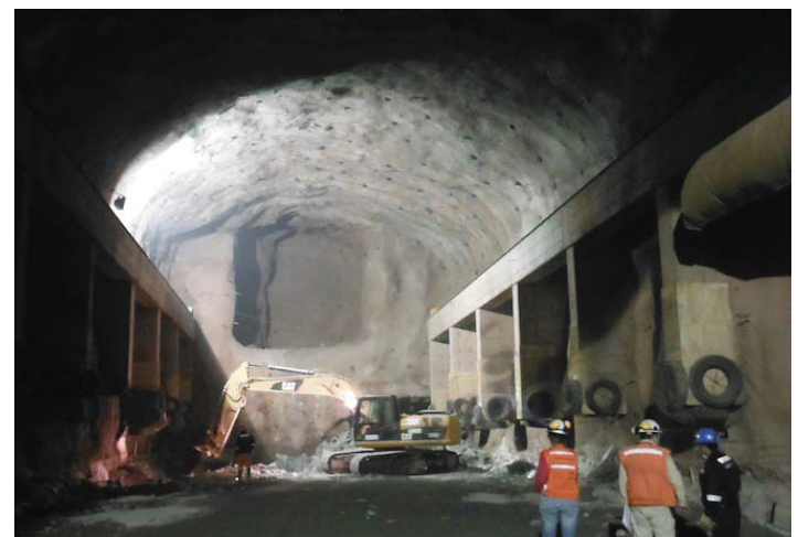
Figure 2. Powerhouse cavern with crane beam.
