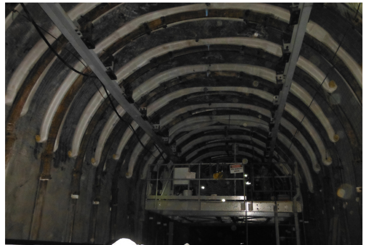
Figure 2. Yielding Steel sets with Bullflex hoses Installation during Tunnel Rehabilitation
