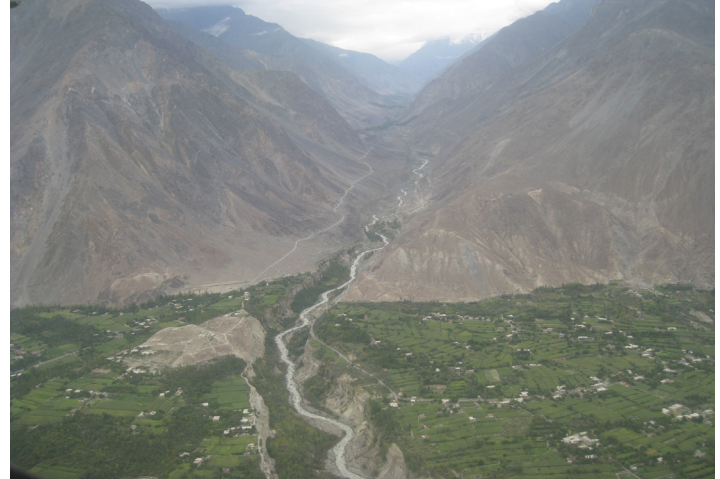
Figure 1. Powerhouse tailrace area.
