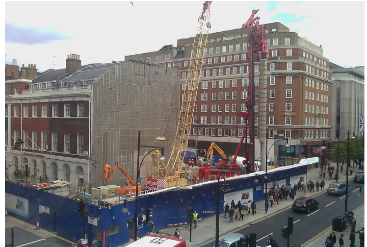
Figure 1. Preparation for new pile foundations for new over-site-development.
