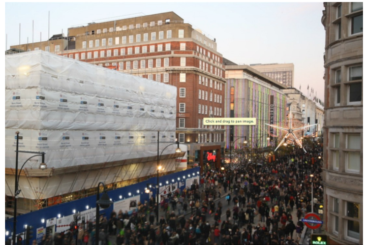
Figure 2. Demolition of one building above station to gain access to construction.
