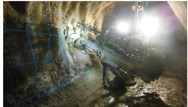
Figure 2. Bingham Drainage Tunnel Excavation.
