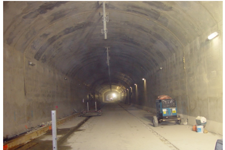
Figure 2. Final tunnel lining in place and finishing out.
