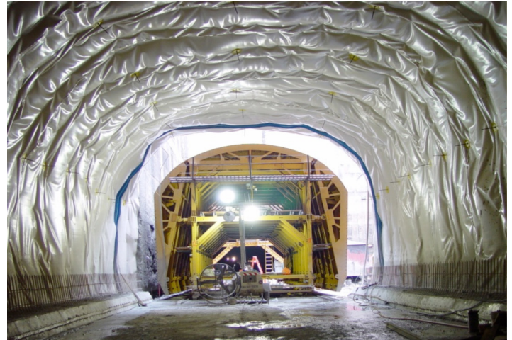
Figure 1. Waterproofing installed, final lining installation ongoing.
