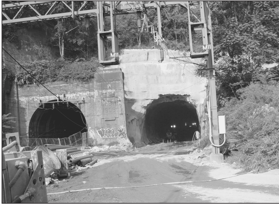
Figure 2. Situation at the East Portal after backfill and tunnel lining removal
