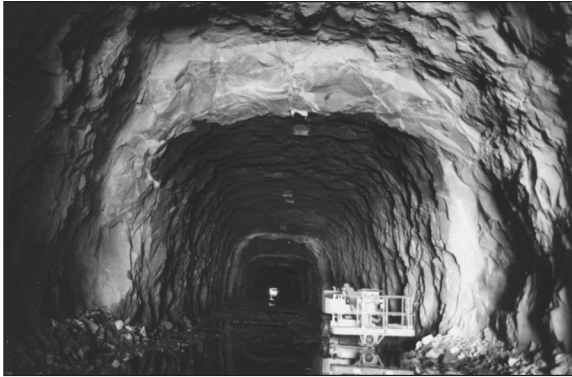
Figure 4. Typical tunnel profile after excavation
