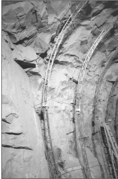
Figure 5. Over break in tunnel shoulder area
