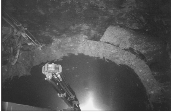
Figure 3. Backfill material behind brick lining
