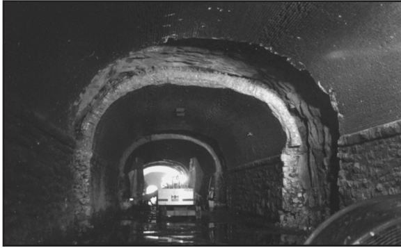
Figure 1. Brick lined tunnel before rehabilitation
