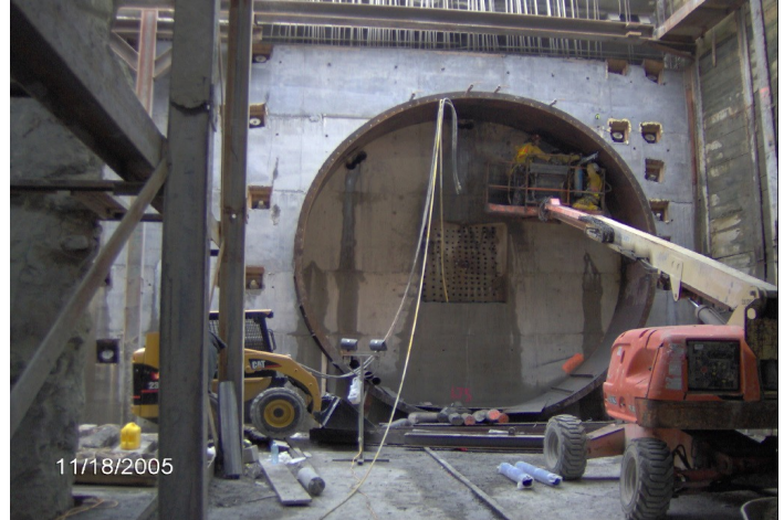
Figure 1. View of West Portal cut and break-out eye for the TBM.
