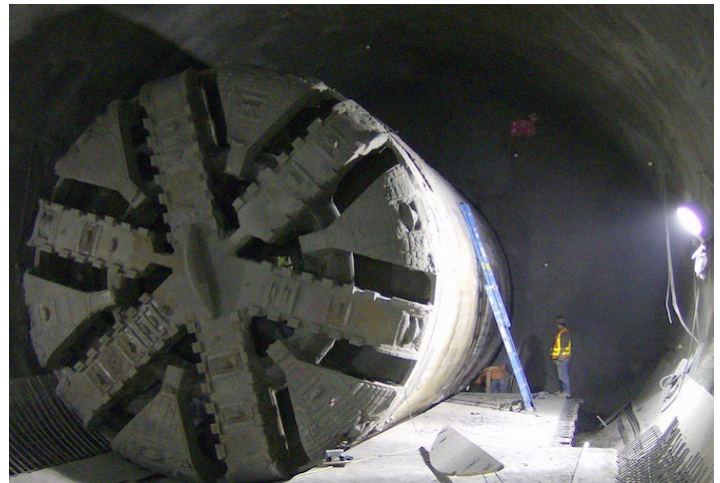
Figure 2. TBM walk-through within the station tunnel.
