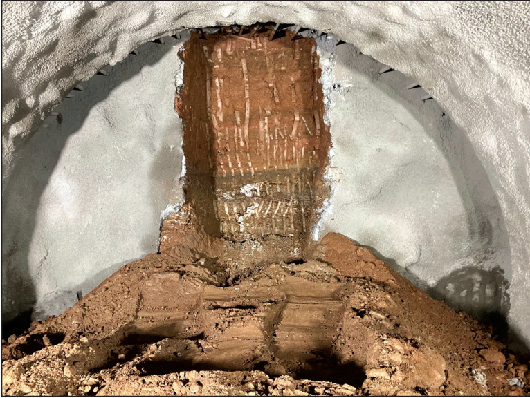
Figure 8. Pocket excavation in soft ground with spiles installed
