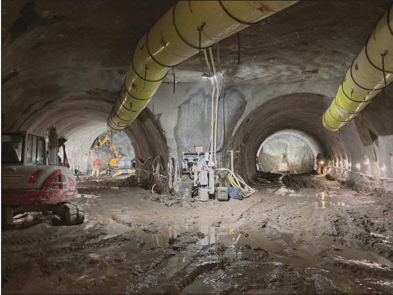
Figure 5. Excavation of the bifurcation
