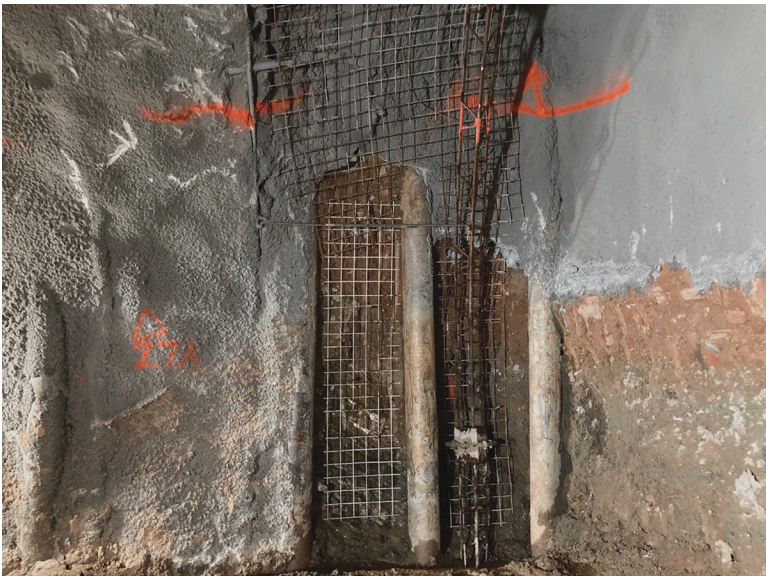
Figure 6. Exposed micropiles
