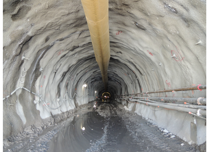
Figure 1. Drill & Blast VA4 heading of the Alfalfal II tunnel
