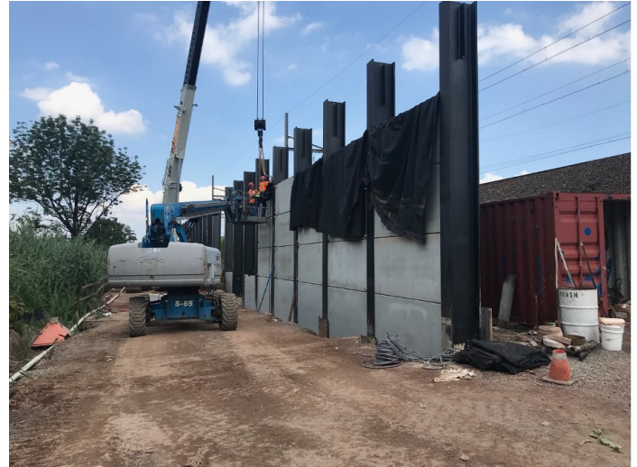
Figure 1. Retaining wall E with soldier piles and precast concrete panels.
