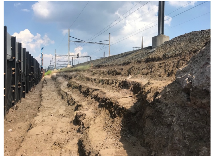
Figure 2. Benches excavated for retaining wall E for subsequent installation of pervious cellular concrete fill.
