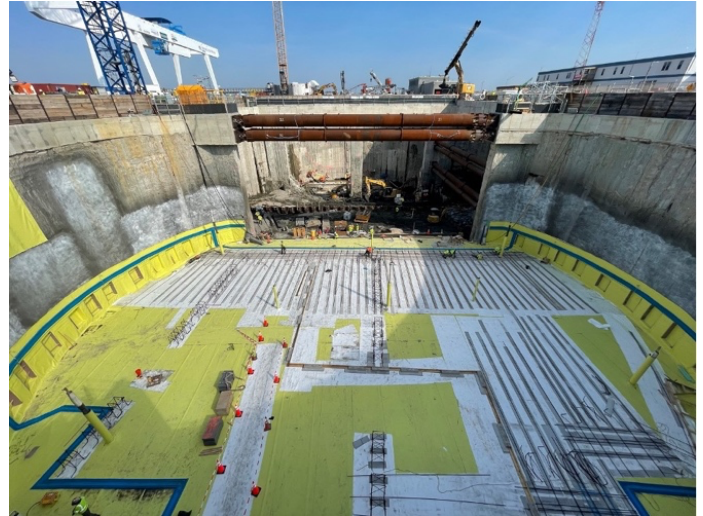
Figure 1. Finalizing installation of waterproofing membrane for the 7-foot base slab. Start of rebar installation in Cell 3 of the South Island Launch Pit.
